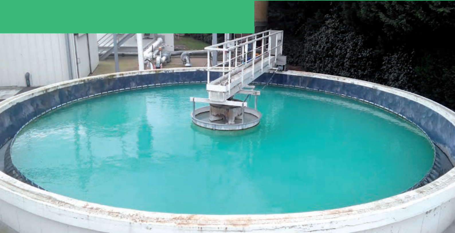
Wastewater treatment plant, ST Tours, France
